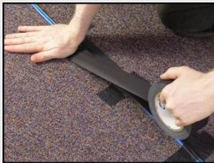
1. Begin by tacking down the cables. Tear off pieces of gaffer's tape and place the strips of tape perpendicular to the cable run about 5 ft (1.5 m) apart.
